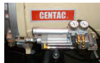
Fig. 13: Inlet guide vane and actuator
